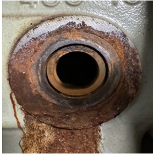
Fig. 2 The part of leakage
