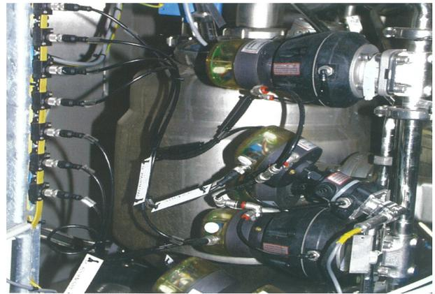
Fig. 7 Simple valve connection on the AS-Interface string
