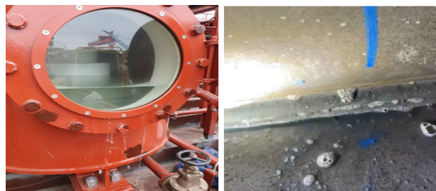
(b) Leakage check by visual inspection
