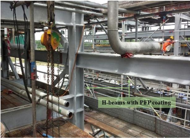
Fig. 1 Structure members with PFP applied (SR group of company, 2021)
