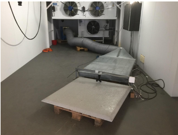
Fig. 8 Cold room facility of GMC for winterization test(URL: http://www.gmc.no )
