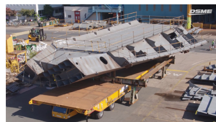
Fig. 1 Transporter and working block (source : DSME youtube channel)
