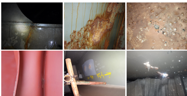
Fig. 1 Hull failure images; crack(top left), corrosion(top middle), pitting(top right), deformation(bottom left), indent(bottom middle), others(bottom right)
