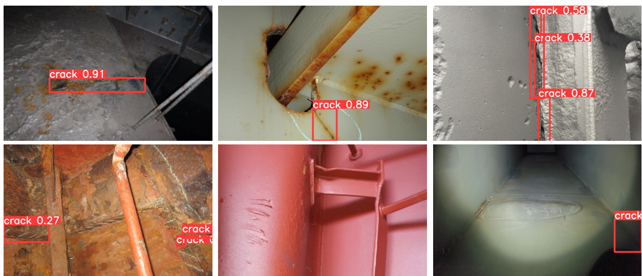
Fig. 11 AI inference at the inspection site: crack(top), another hull failure(corrosion, deformation, indent)(bottom)
