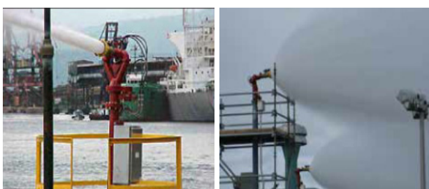
Fig. 1 Installation of fire fighting monitor
