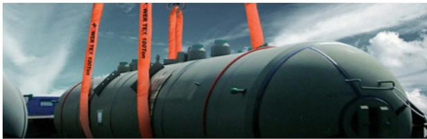
(a) Sling belt for lifting a tank
