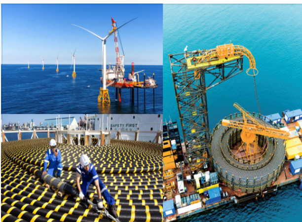
Fig. 2 Installation of dynamic power cable(LS전선)
