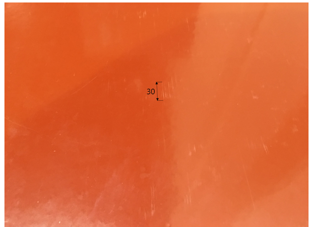
Fig. 6 Coating condition after the phase 1
