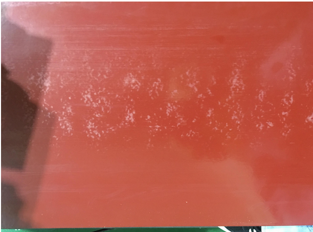
Fig. 9 Coating condition after the phase 4
