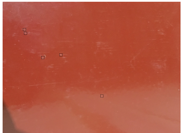
Fig. 7 Coating condition after the phase 2
