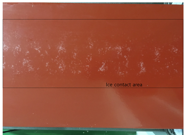
Fig. 8 Coating condition after the phase 3
